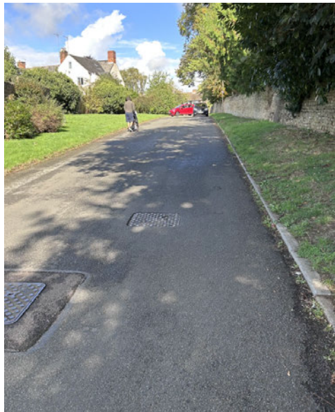
Fig 5 – Painters Close, note the lack of any pavement or streetlighting.
